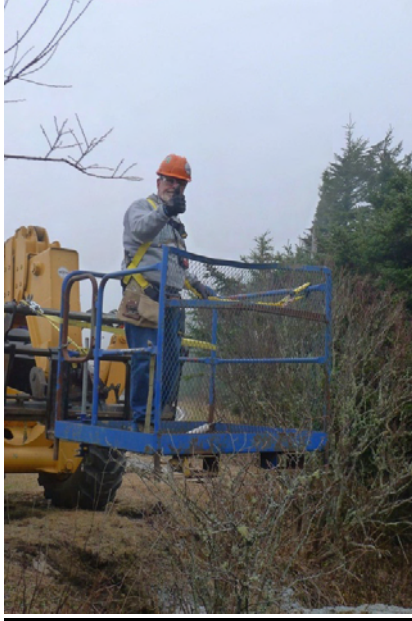
John prepares to mount the transmitter antenna onto the tower
